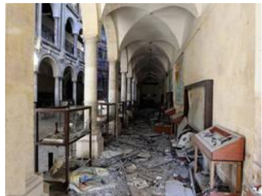
Example of damaged site in Syria
